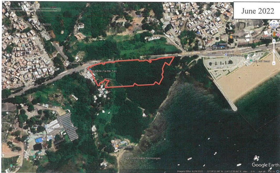
Figure 1-2 According to the aerial photos from Google Earth, the application site (marked in red) has been subject to land formation and vegetation clearance since 2024
